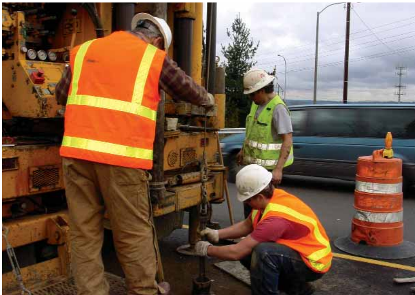
The Everett Project will greatly improve traffic flow in one of I-5's major bottlenecks.
