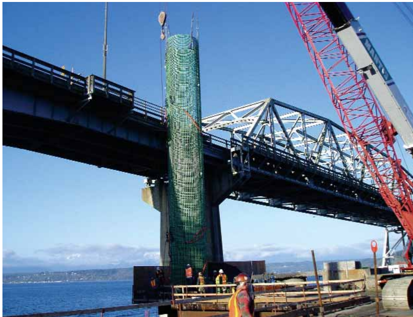
On the other side of Puget Sound, the Hood Canal Bridge project will greatly improve safety and add another traffic lane to the bridge.
