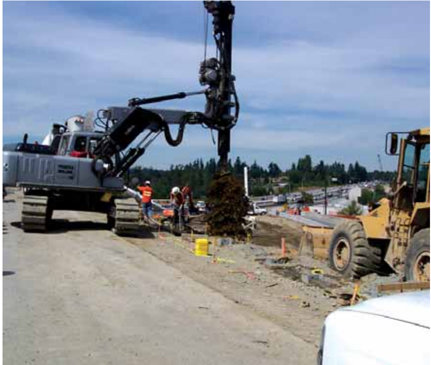
Oregon and Washington are both using design build contracts to help speed up construction.
