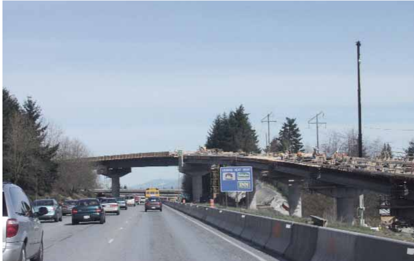
The flyover will improve traffic mobility near Everett.
