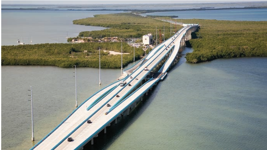
The Florida Dept. of Transportation will be making extensive use of design-build for its stimulus projects. (Photo courtesy Granite Construction Co.)
